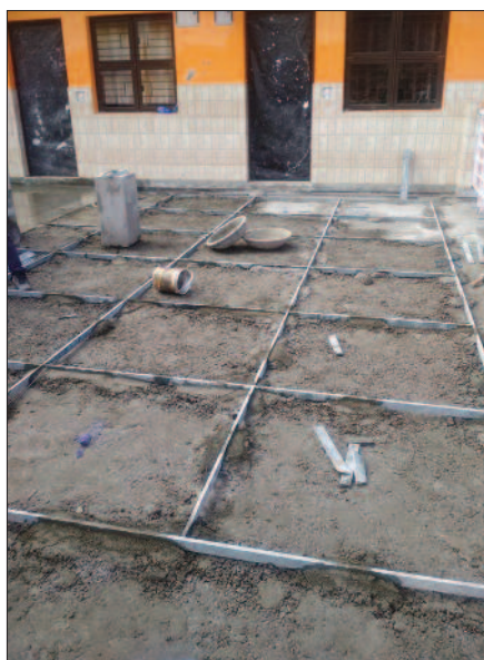
Construction of waterproof walkway.
